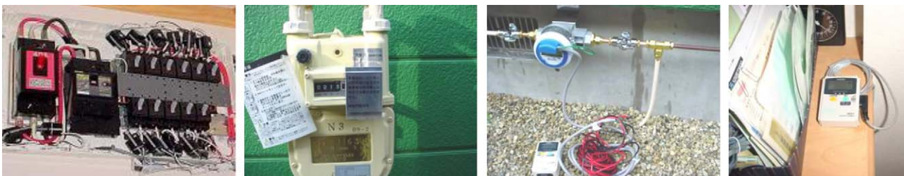
Fig. 2. Measuring instruments (from left to right: electricity, gas, kerosene and air temperature).
